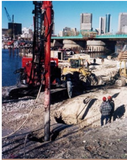
A PTC Vibrolance is installing 5 lines of 10 m depth stone columns on 2 km along the river banks of the Red River, Winnipeg, Canada.
