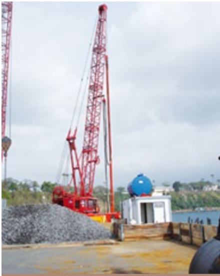
Two Vibrolances doing top feed stone columns under water at 17m depth for the Malabo Harbor, Equatorial Guinea.
