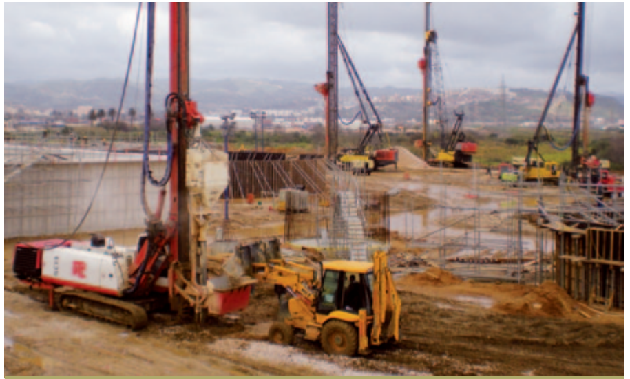
The SC13 and 3 sets of VL18 BFS Vibrolances installing 6500 stone columns for the extension of an oil refinery at Skikda, Algeria.
