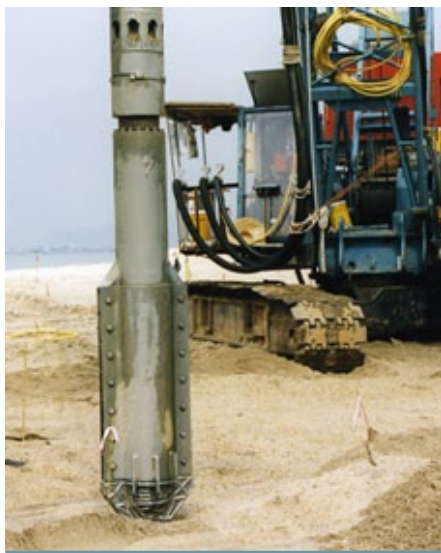
Vibrolance VL110 working at 31m depth to compact 2.000.000 m 3 of land reclamation for the extension of the LAMME power station, Hong Kong.
