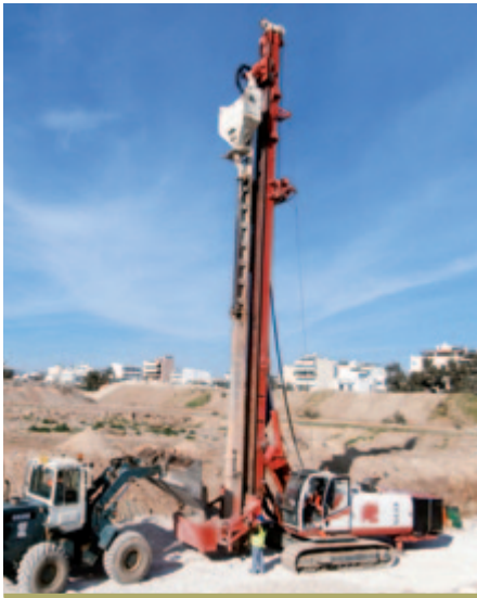
The PTC SC13 installing 1500 stone columns of 11.5 m depth and 800 mm diameter for a new cultural center in the city of Athens, Greece.
